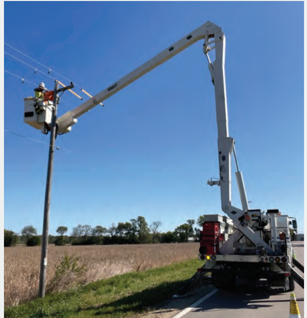
Pictured: Apprentice Lineworker Paul replacing an insulator. Photo courtesy of Michael Nawrocki.
