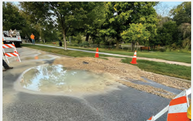
Pictured: Result of a water main break on Division Street. Photo courtesy of Kent Thompson.
