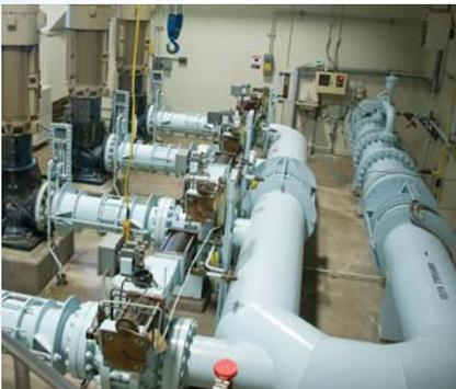
**Wastewater Treatment Plant** - This locally-owned public power utility made several upgrades at their plant and used RFP funding to install a high-efficiency blower with a variable frequency drive, as well as additional aeration piping and blower control system upgrades. These energy efficient upgrades made it possible to reduce expenses, better serve ratepayers, and run the wastewater treatment plant more effectively.
