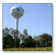
Stoughton has two water towers totaling a combined 900,000 gallons of water storage. Water is pumped from one of the city's four wells into these water towers where it is stored until you turn on a faucet or flush a toilet. The pressure from the water in these elevated water towers helps push the water through the distribution system and into your home.
